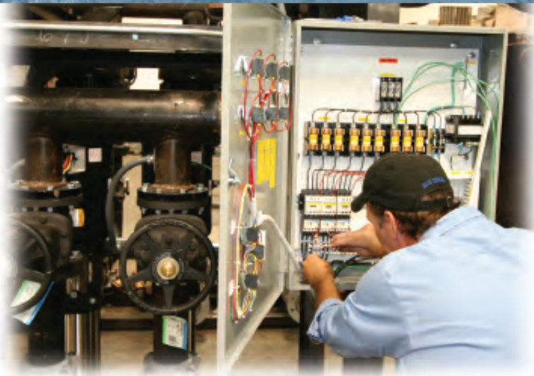
Wiring a Class "S" Deaerator
