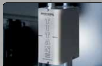
AUXILIARY LOW WATER CUT-OUT
