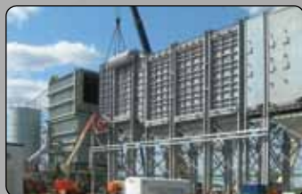
Erosive and corrosive resistant solid fuel (coal-fired) HRSG.
