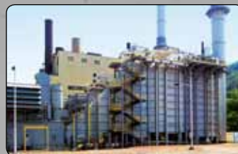
Modular designed, field-erected utility combined cycle HRSG.
