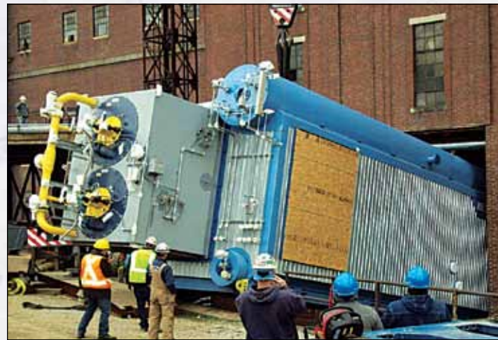
A pair of 220,000 PPH watertube boilers being delivered to Canada on special "perimeter-frame" trailers.
