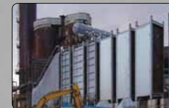
A 450K PPH waste heat recovery project, expected to produce upwards of 40 megawatts.
