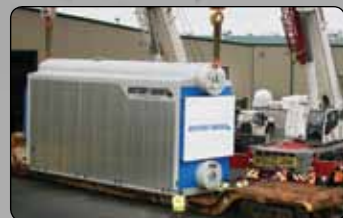
Load-out of "O" type WHB designed to produce 100,000 PPH of super heated steam at 850 PSIG/824°F.
